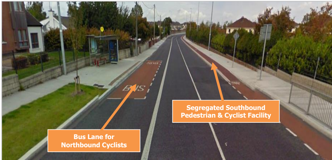
Figure 3.4: Cycling Facilities on Ballycullen Road
