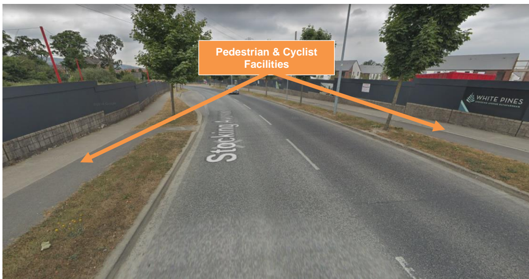
Figure 3.2: Pedestrian/Cycle Facilities on Stocking Avenue Looking West
