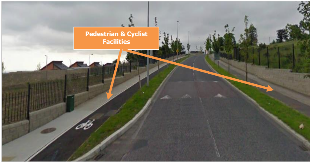
Figure 3.3: Stocking Avenue Looking East
